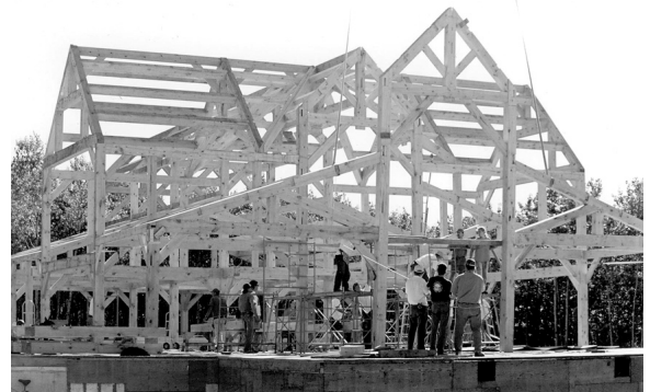
The raising of the timber frame beams, called bents, July, 1999
